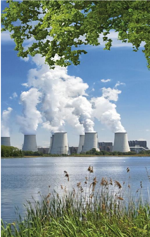
Flue Gas Cleaning
