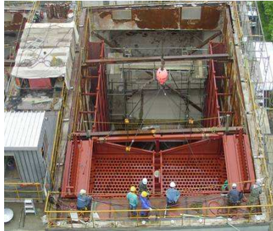
Bag plate under construction
