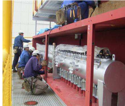
Pressure tank under construction
